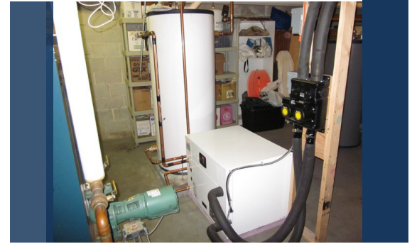
Bosch TW036 water-to-water system provides domestic hot water
