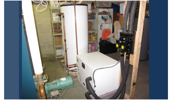
Bosch TW036 water-to-water system provides domestic hot water
